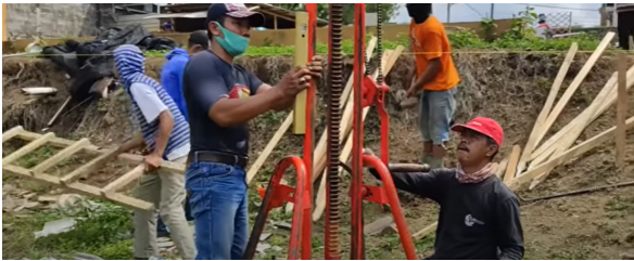
Gambar 3 Persiapan sondir
